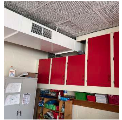
Original 1958 classroom casework
