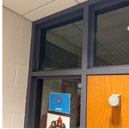
Wire glazing at classroom doorway
