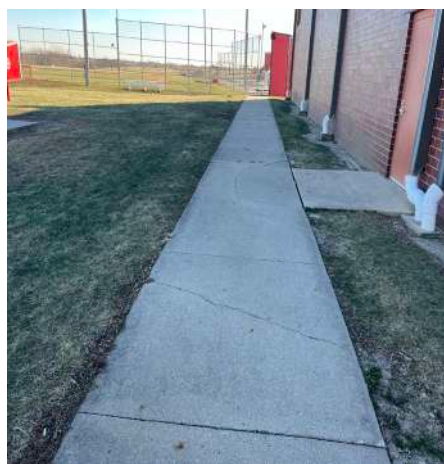
Concrete sidewalk in fair condition.
