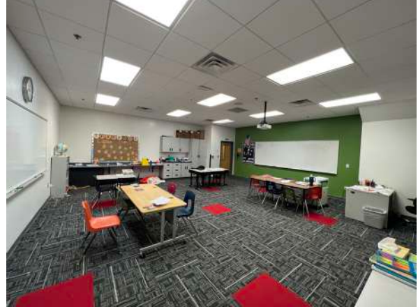
New carpet tile (recently installed due to water damage)
