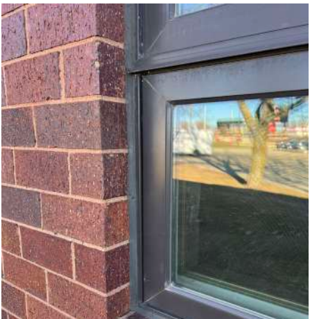
Window caulking in fair to good condition
