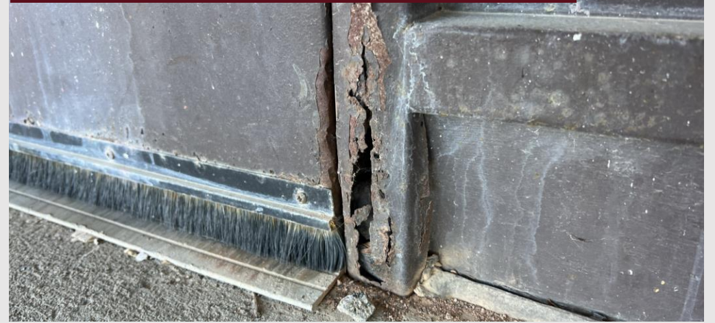
CURRENT CONDITION OF JR/SR HIGH VESTIBULE DOORS
